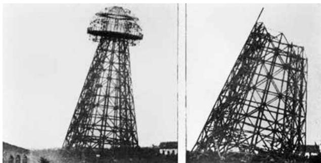
Figure 3. Photo of the partial demolition of the tower at Wardencllyffe, July 1917. Initial dynamite blasts failed to bring the tower down; it took until September 1917 to raze it completely. *The Literary Digest* 55, no. 8 (1917): 25.
