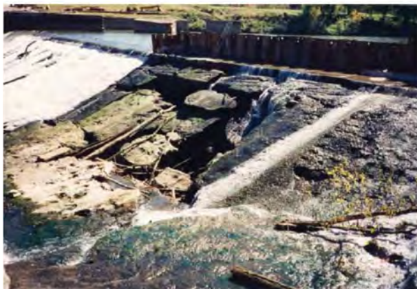
Figure 3. Left photo shows the collapsed portion of the dam near the left abutment in 1994. Right photo shows dye leakage at the left abutment in 2001 (Welshans et al., 2011).
