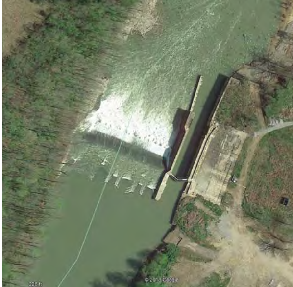
Figure 2. Aerial view to the northeast (upstream) of Dam 8 on the Kentucky River as of 2017 showing the completed concrete-filled cellular sheet pile structure.
