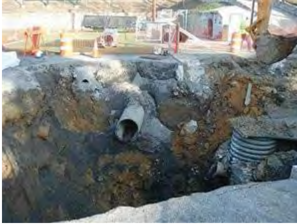
Figure 3. Excavation of the subsiding reinforced concrete manhole in April 2013. Note the 0.5 meter diameter pipes feeding the manhole.
