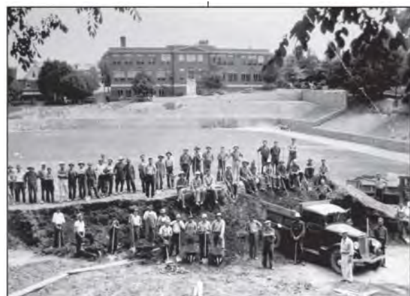
Figure 2. Works Project Administration workers during the construction of Memorial Field, circa 1937. View of the stadium to the south (from Smith, 2011).
