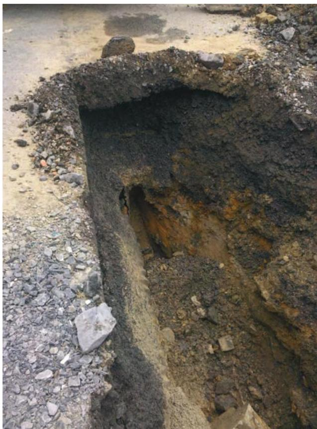
Figure 3. Fracture discovered during grading operations. Note the iron staining on the wall of the fracture.
