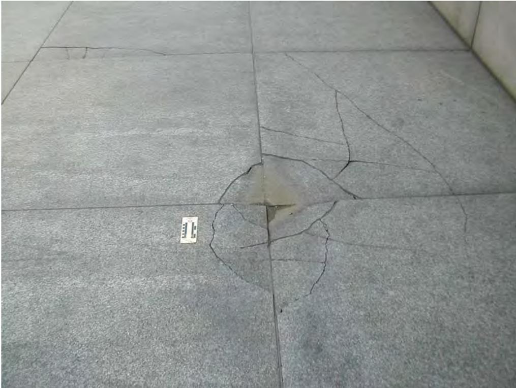
Figure 2: Deformation of the expensive granite pavers due to subsidence of the fill materials (plastic scale is 1 foot).
